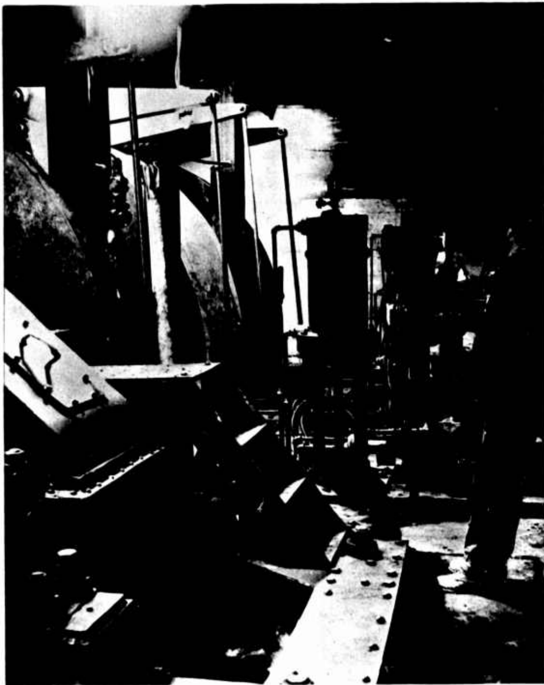
FIG. 3. Hoisting Equipment With Hydraulic and Electro-mechanical Controls. Located 470 feet below the sea level and approximately 400 feet below the sea floor (Dominion Coal).
